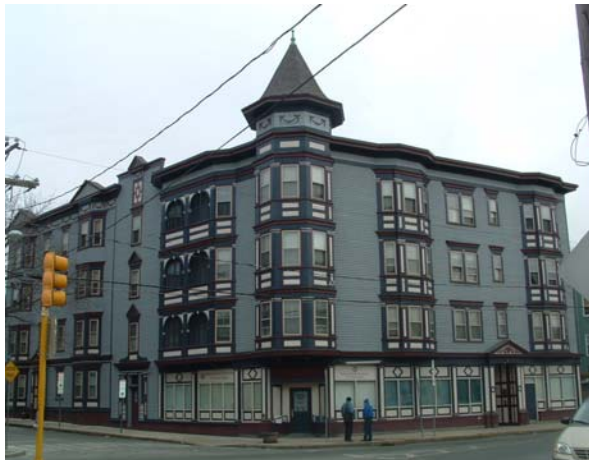
The Bow Street Apartments include 18 affordable rental units with two to four bedrooms on the upper floors and retail space on the first floor, currently used by the Mt. Auburn Hospital Clinic. This project was a substantial rehab of a historic building constructed in the late 1800s. Source: Somerville Community Development Corporation
