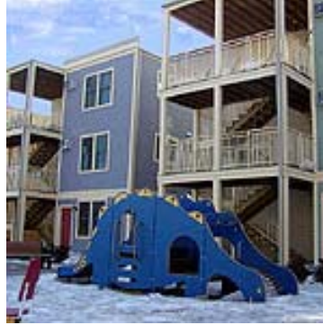
The Linden Street Apartments include seven buildings and 42 affordable rental units. The project used Low-Income Housing Tax Credits and was built on a brownfields site. It has won green building awards and has been recognized nationally for its sustainability efforts. There is a common green and tot lot in the center of the development, and each unit has a private porch that overlooks the common areas. Source: Somerville Community Development Corporation
